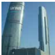
UAE, Abu Dhabi, Sun and Sky Towers Al Reem Island Luxury residential buildings Simplebus TOP and CCTV System 1104 Planux
