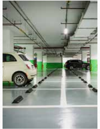
CHECKING ON CAR PARKS
