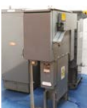
DSS G Packaged Substation Merlin Gerin SE6 630A Switch + Transformer Earth Switch
